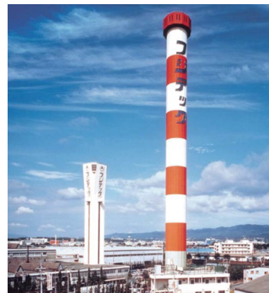
150-meter elevator research tower, tallest and largest in the world*(1975)
