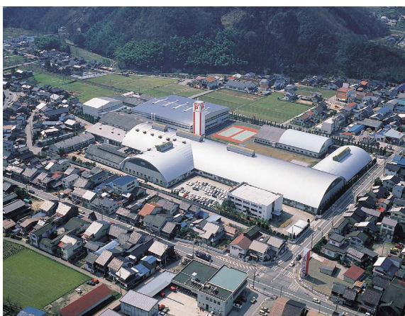
The "Hidaka Plant," went into full-scale operation (in February 1990).
